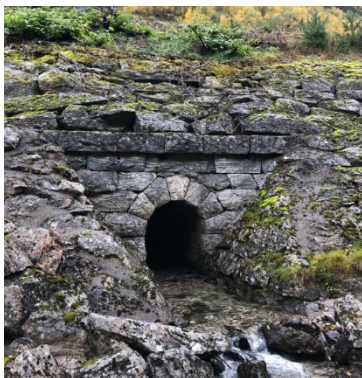
Figur 3-10 Kverngrova kulvert. (Foto: Asplan Viak, 2024).
